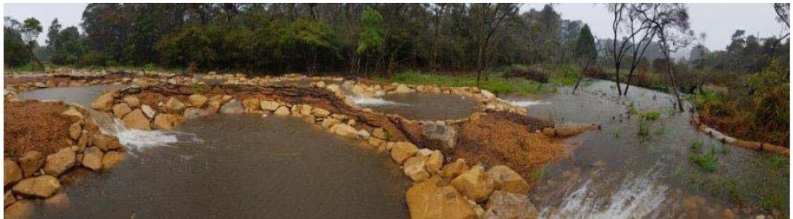
Figure 2: Central Park raingardens in flow
